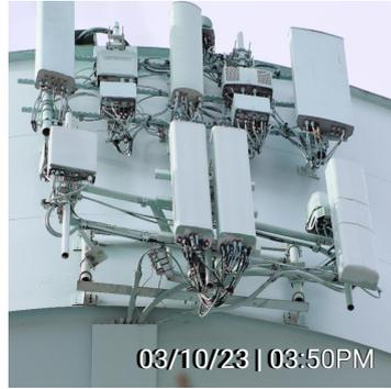
9. Cell group 3 - Spectrum major equipment removed except the antenna mount. Paint color doesn't match
